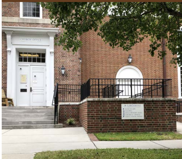
The Monroe Place entry steps and ADA-compliant ramp funded by the estate of Richard Norman.
